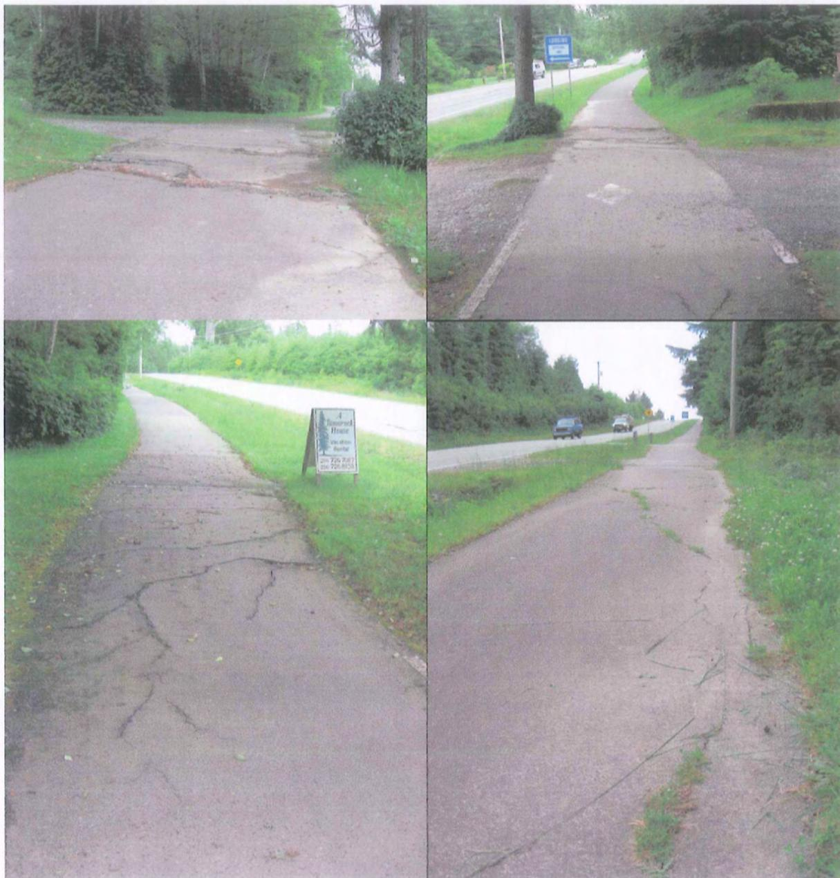
**Bike Path Pavement Damage – tree roots that have lifted pavement surface creating hazards.
